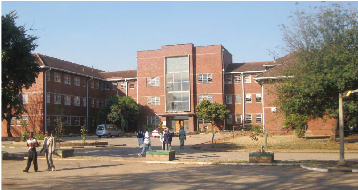
Second Level Hospital
